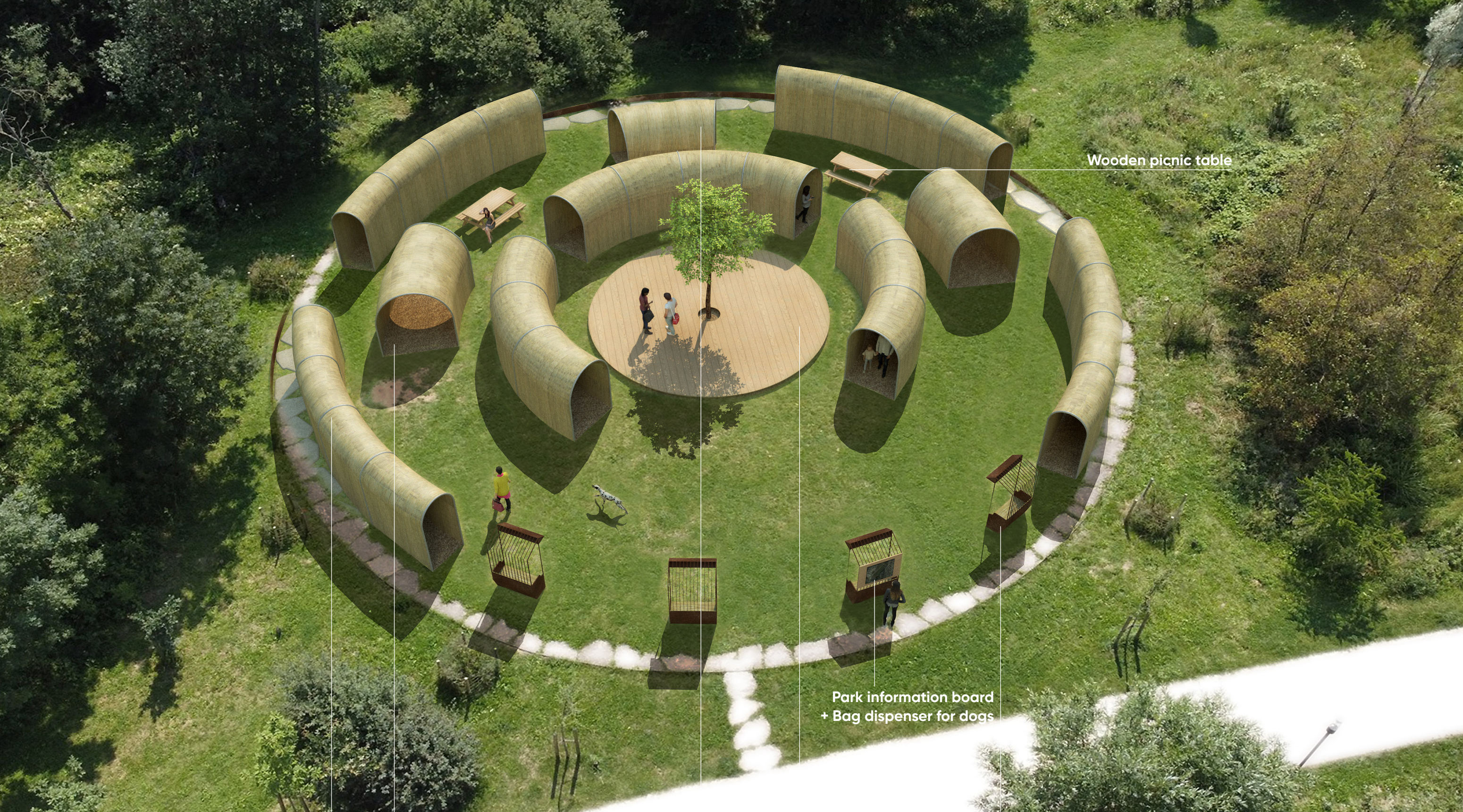
Structure of the tunnels in galvanized steel arches + Flexible steel strip supporting reed rollers
